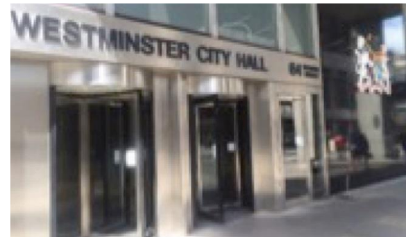
£80m City Hall refurbishment
